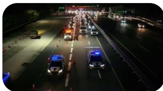
Peningkatan Keselamatan lajur Contra Flow Pemasangan water barrier tiap 50m, LED clip, pace car , dan Lane Control Signal (LCS)
